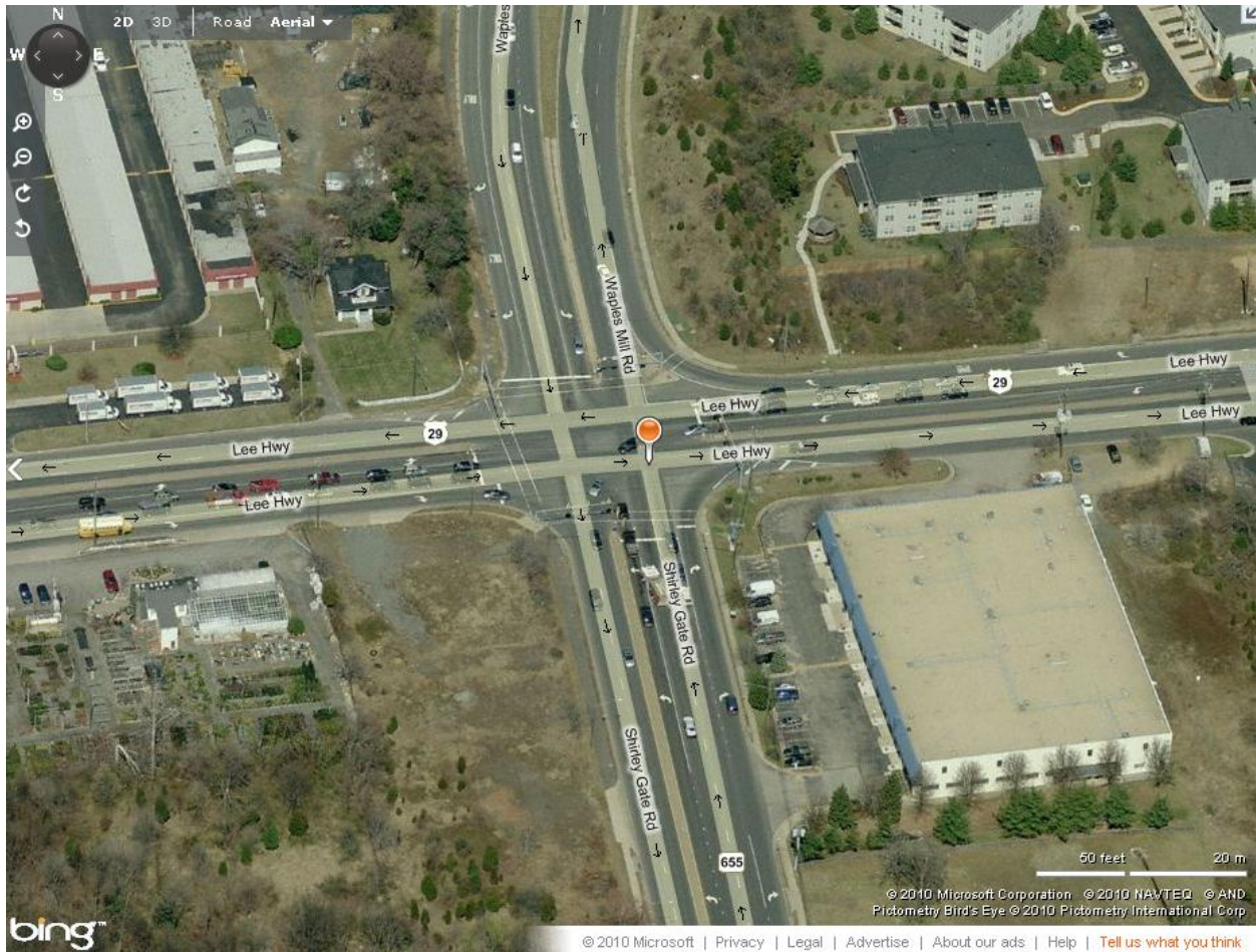
Figure 8. Aerial Image. Lee Hwy at Waples Mill Rd and Shirley Gate Rd (node 277764). This intersection served as a high-crash intersection in the analysis. (Source: www.bing.com , 2010)
