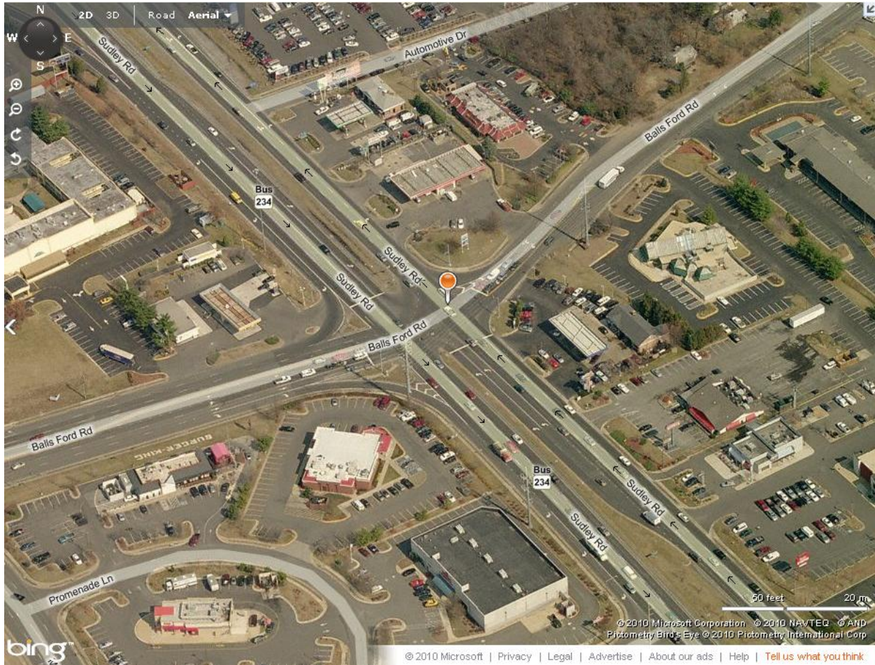
Figure 10. Aerial Image. Balls Ford Rd at Sudley Rd. This intersection served as a low-crash intersection during analysis. (Source: www.bing.com, 2010)
