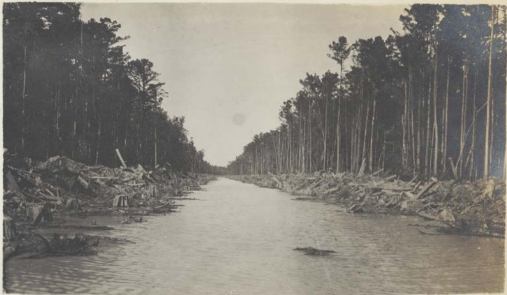
Ditch 85 Looking north from Sta. 84.
