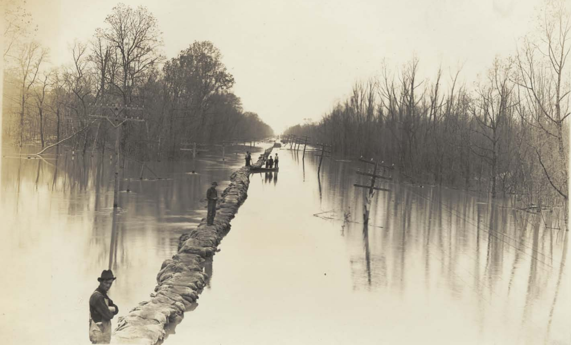
TWO AND ONE-HALF MILES NORTH OF BRIDGE JCT., ARK. LOOKING NORTH TOWARDS MARION
