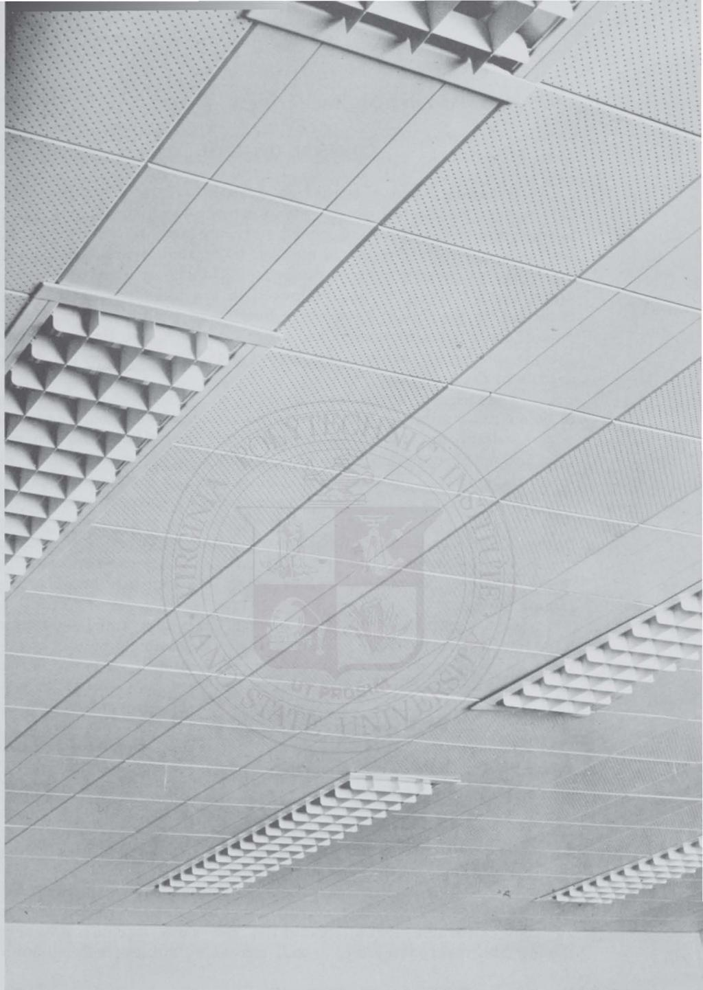
Figure 51. Completed Ceiling Showing Electrical Fixtures, Heating Panels and Accoustical Material in Place.
