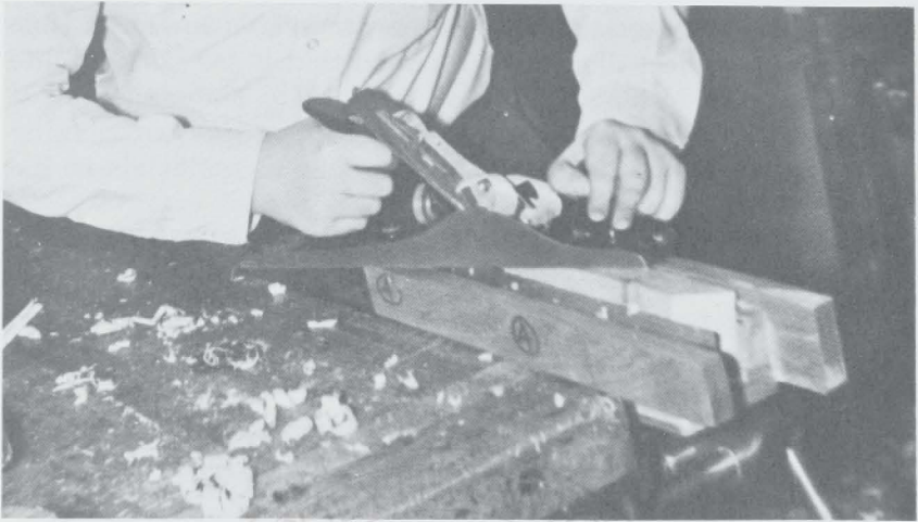
Fig. 6. Planing Fixture in Use
