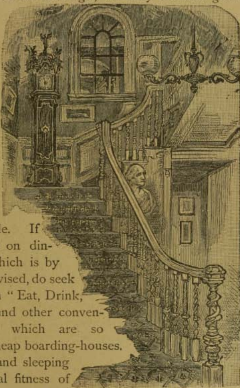
STAIRWAY OF THE LONGFELLOW MANSION.
