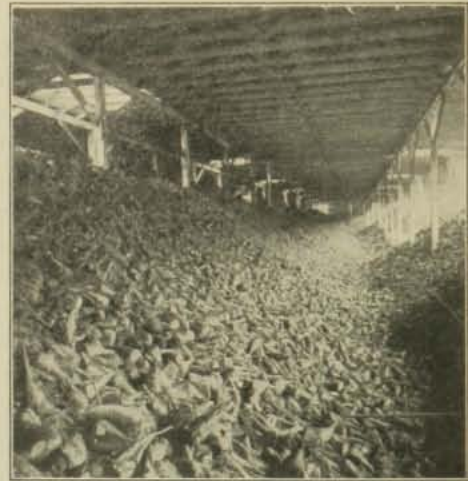
A shed for storing beets—canals under the bins carry the roots to the washing room
