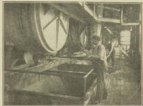
Crystallizers to concentrate the sugar juice
