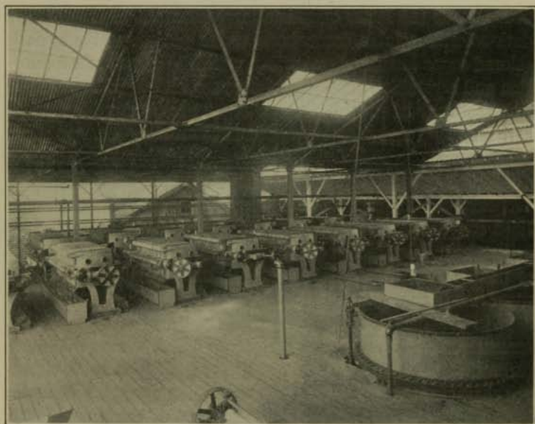
FIG. 31. — Filter presses in sugar factory (American Photo Co., Havana).
