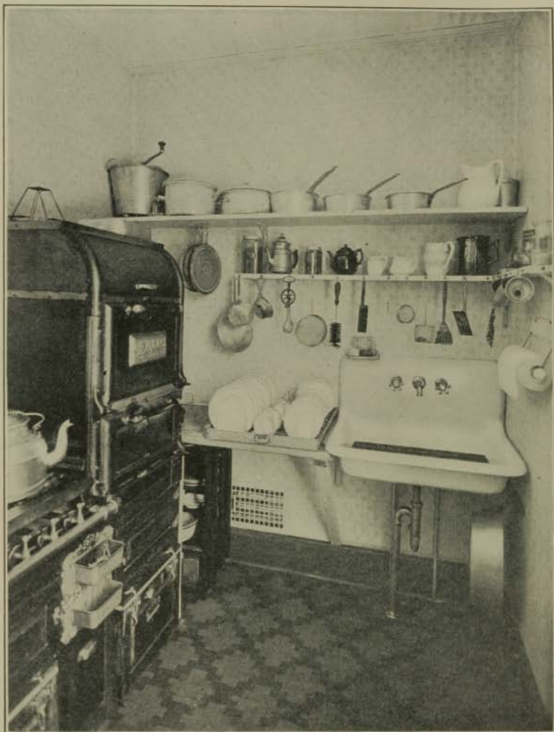
KITCHENETTE WITH GAS-RANGE.
