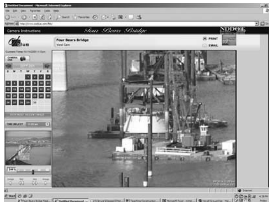
Figure 5: Four Bears Bridge photograph taken 9/30/04 at 11:05 am (Oxblue Corporation, 2005).
