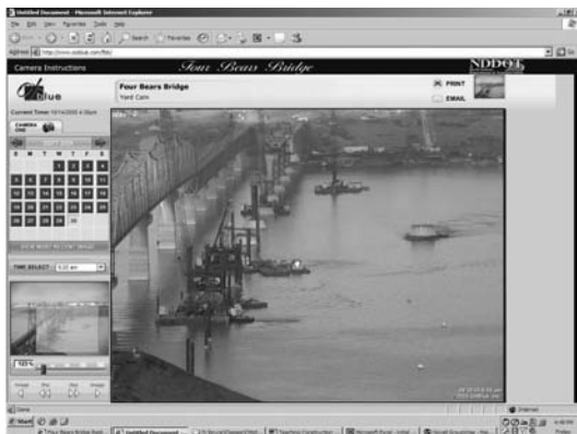
Figure 6: Four Bears Bridge photograph taken 30 September 2004 at 9:10 am (Oxblue Corporation, 2005).
