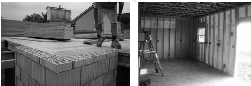
Figure 2. Swiss Masonry Walls (left) and U.S. Wood-frame Walls (right) (photos by authors)
