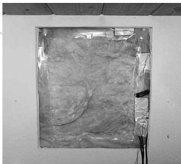
Figure 4. Polyethylene Vapor Retarder, Laramie
