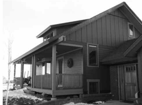
Figure 2. Laramie Test Project
