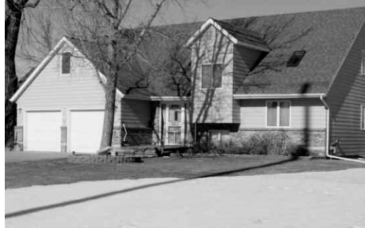
Figure 1. Kearney Test Project
