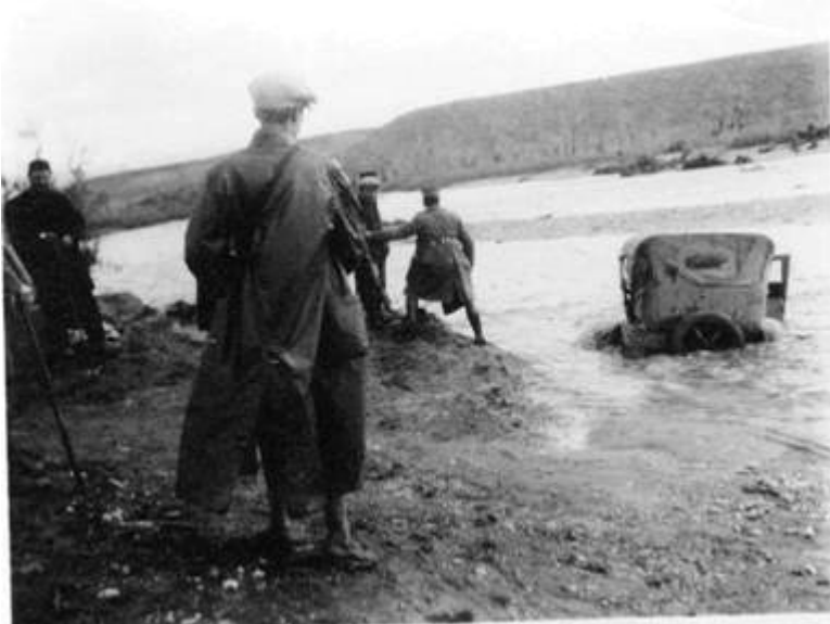
Photograph 1. Fording the River to Olynthus
