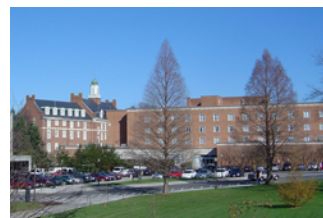
Donaldson Brown, seen here from Kent Street, will become graduate housing and a Graduate Life Center.
